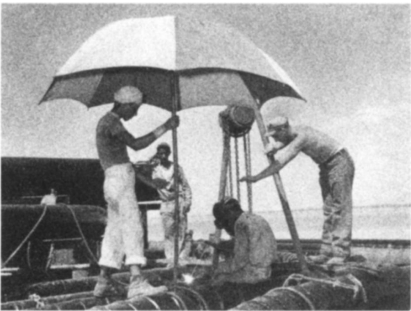
Enclosure for desert welding
